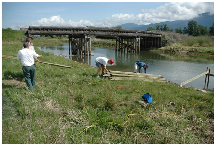
Figure 10: Indian Creek bridge by North Pump inlet (left) and bridge inspection for piling rot October 2005 (right).
