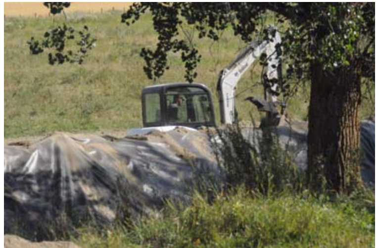
Geotech cloth application
