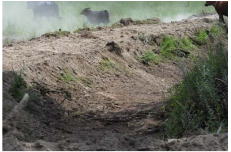
East side canal berm
