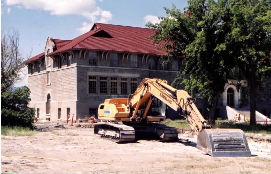
Photo of St. Eugene Mission 2002 – Note entrance to bat roost at roof peak.
