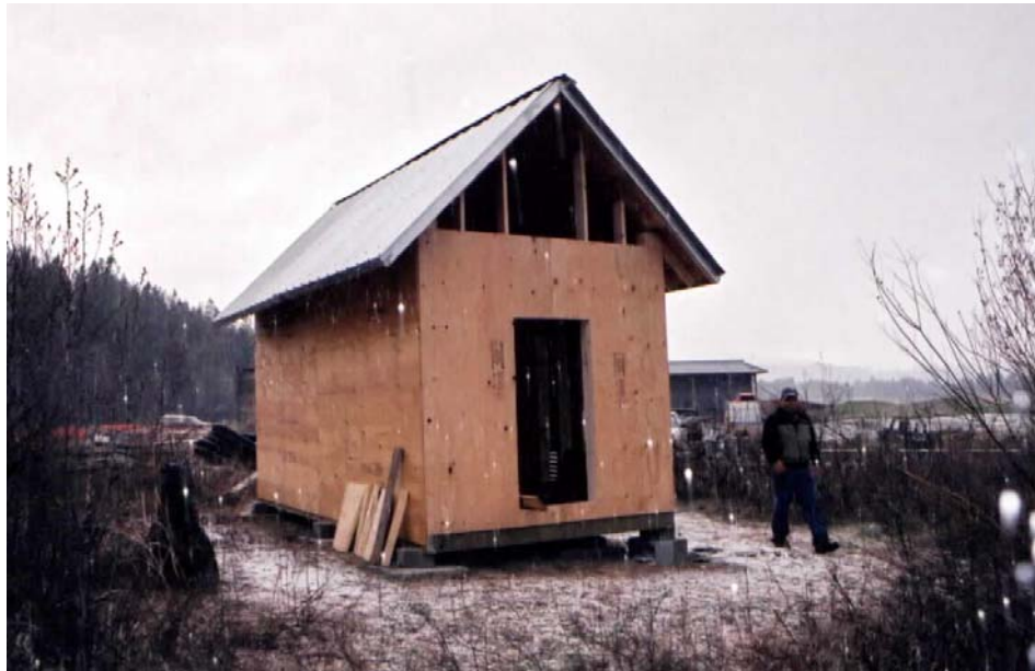
Photo 3. New Roost Structure under Construction.
