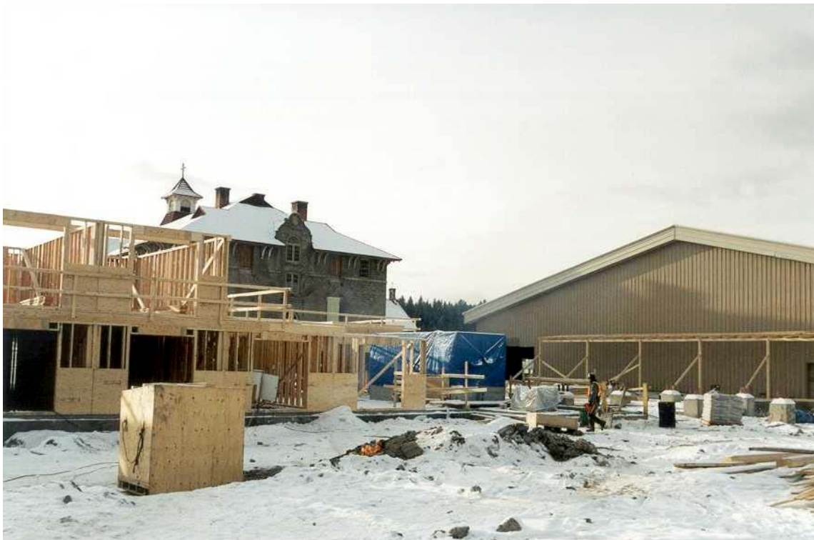
Photo 1. Construction at St. Eugene Mission Winter 2002.
