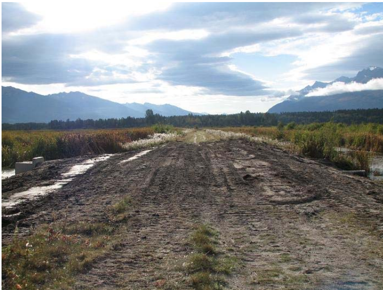
Figure 8. New control and exit pipe installed. Control visible at left side of dyke; outlet pipe visible at right side. Seeding still required (September 2007).
