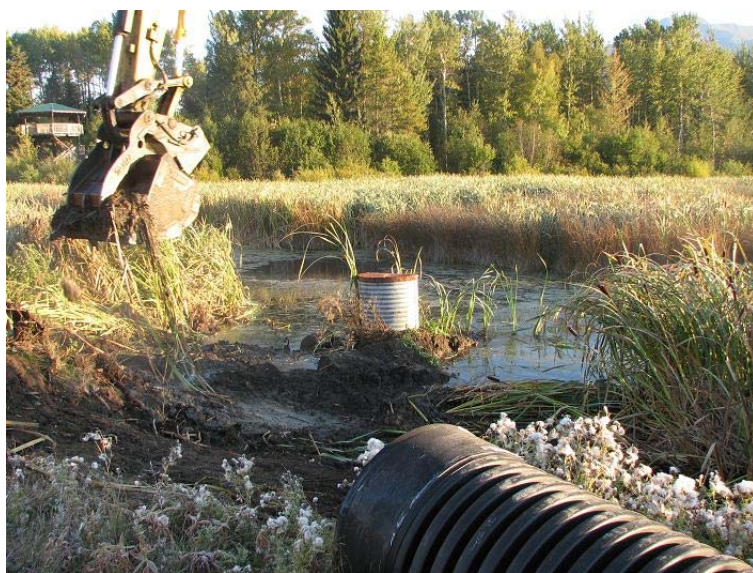
Figure 6. Exposing old control structure (September 2007).
