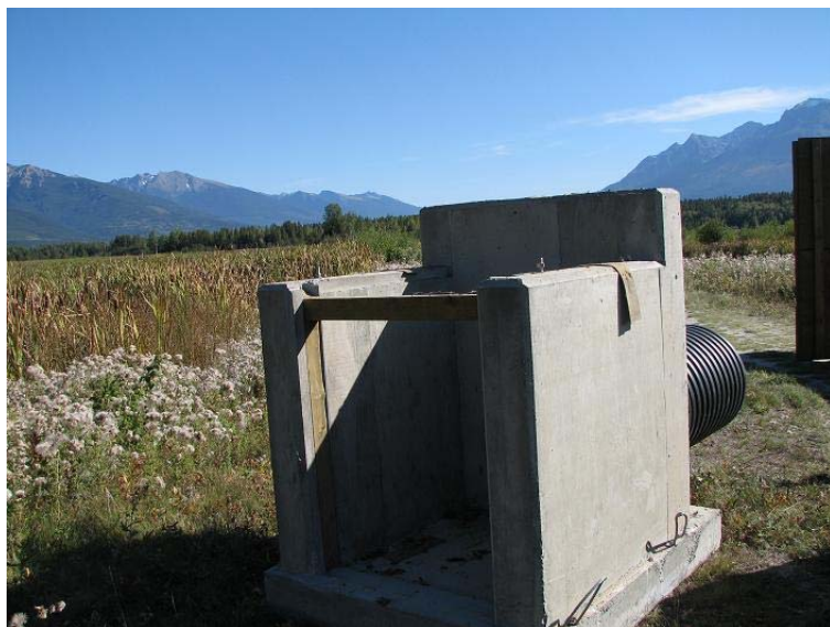
Figure 3. New control structure to be installed (September 2007).
