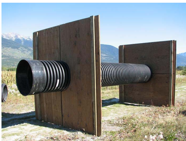
Figure 4. New exit pipe and plywood seepage collars to be installed (September 2007).
